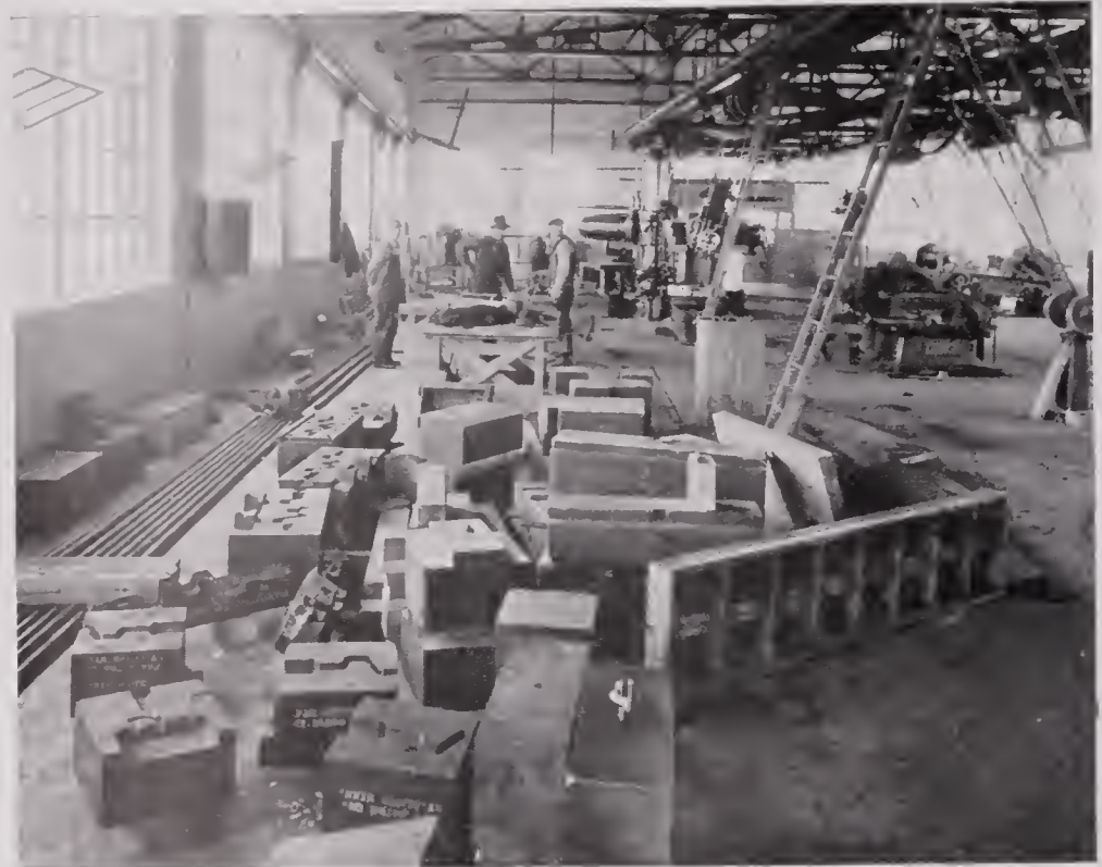
DIES AND TRIMMING BLOCKS
